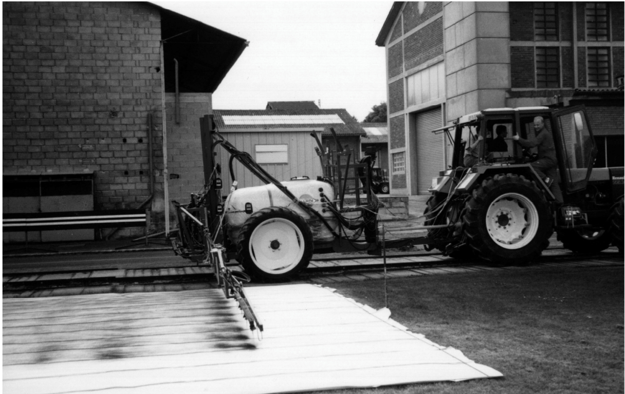
Fig. 2. Experimental test on concrete track
