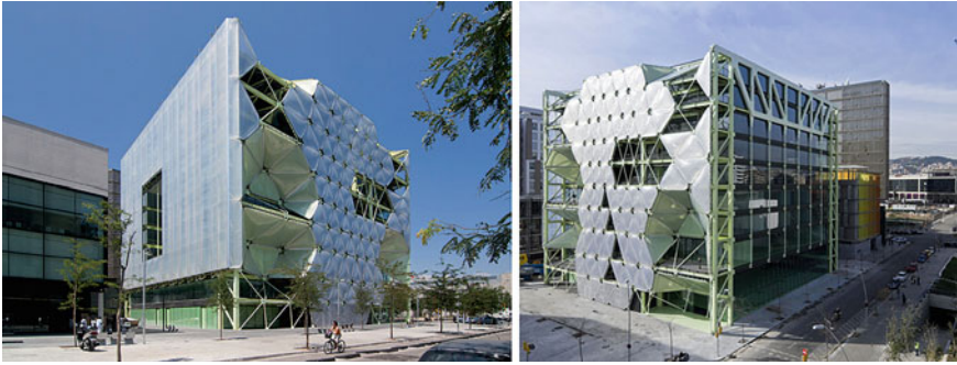
Fig. 1 Views of the Media-TIC building. Left: SE and SW façades; Right: SE and NE façades. Credits: José Miguel Hernandez, Iwan Baan
