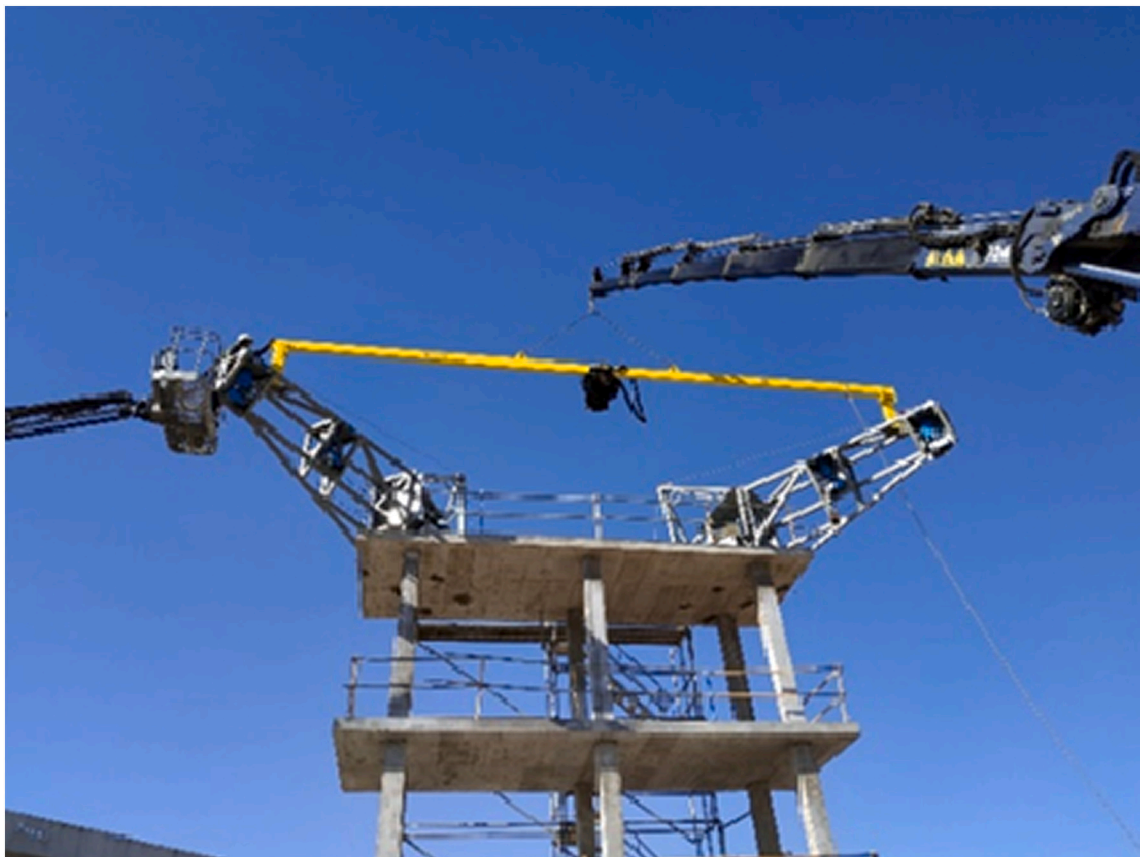
Fig. 23. Fixing supporting structure systems to demonstration building.
