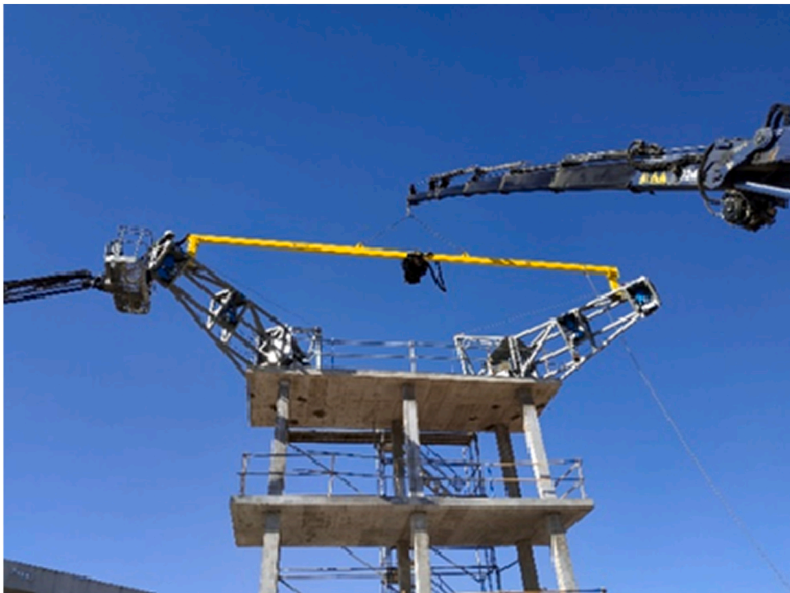
Fig. 23. Fixing supporting structure systems to demonstration building.
