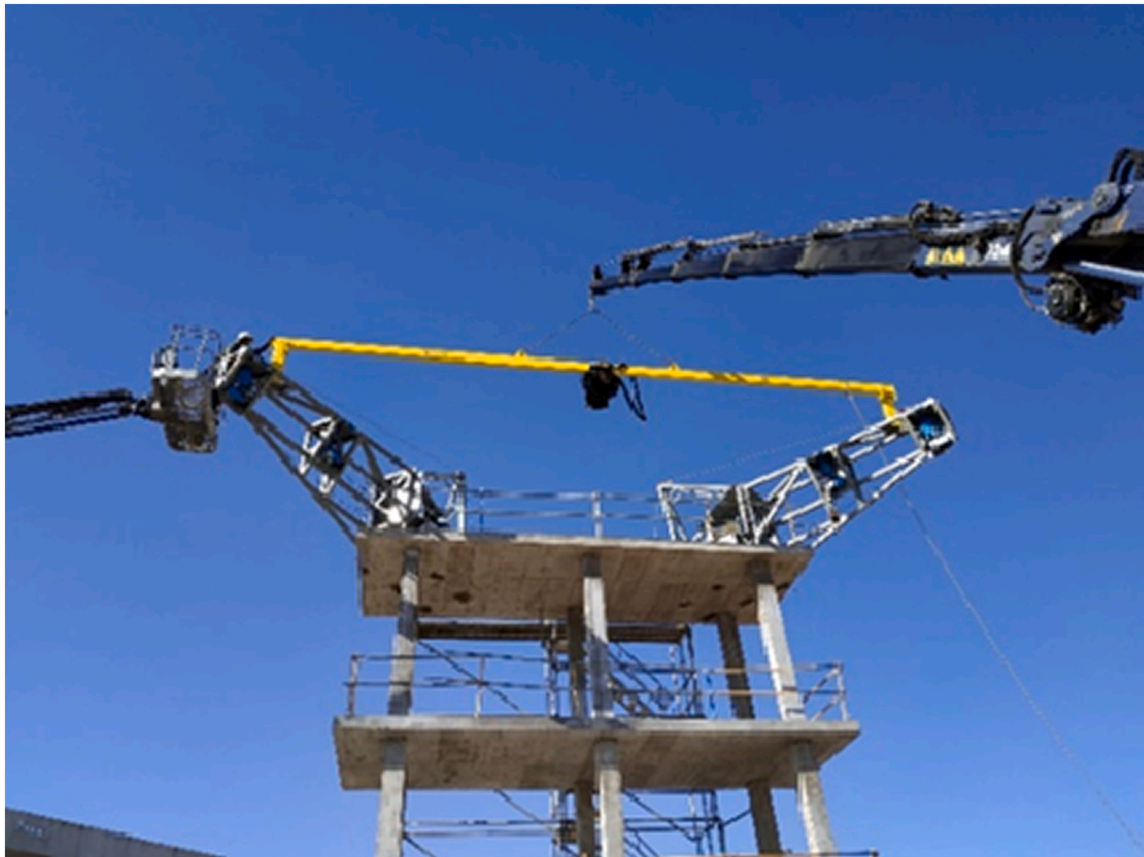
Fig. 23. Fixing supporting structure systems to demonstration building.
